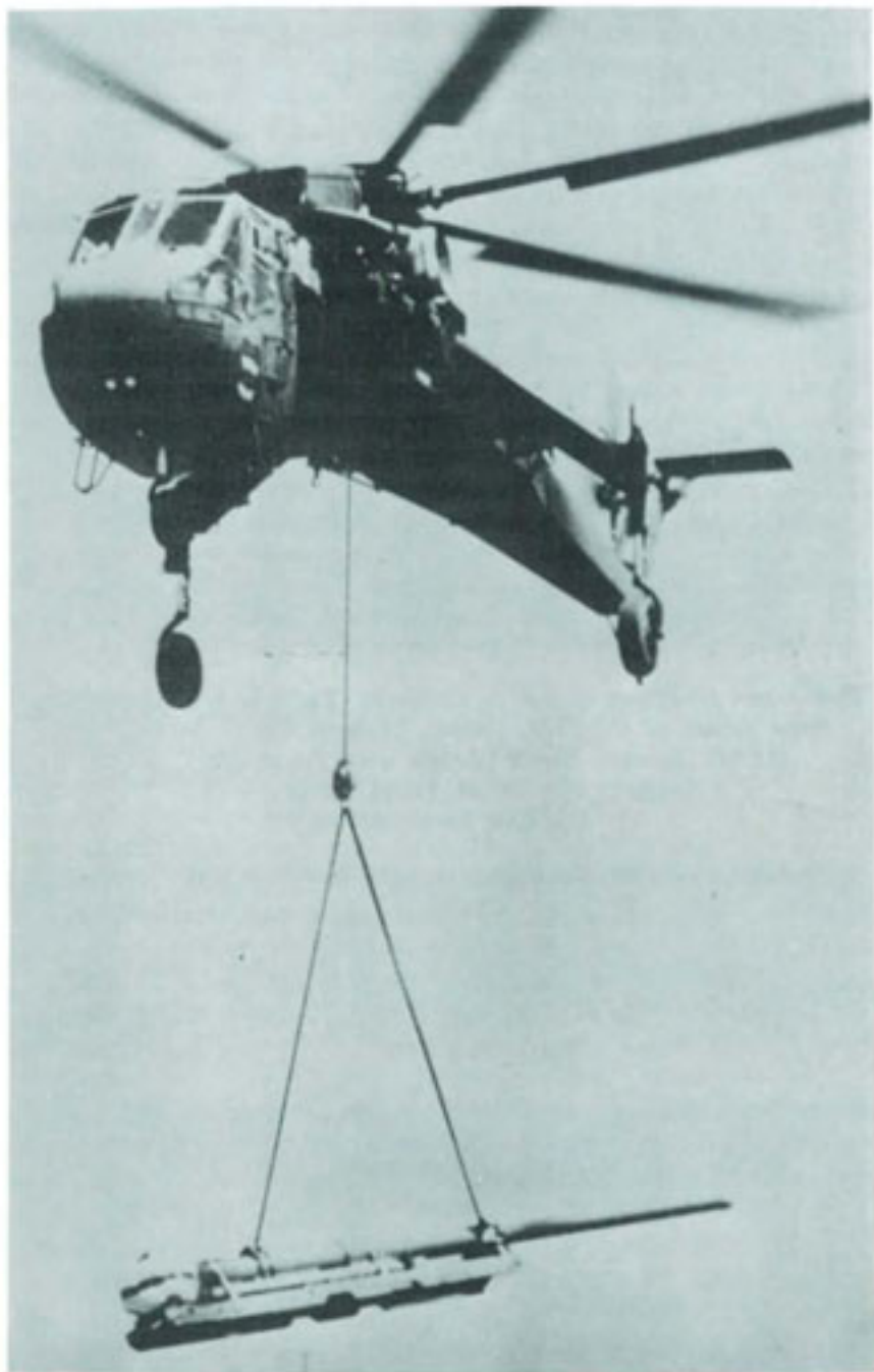
FLYING CRANE LIFTS 175MM GUN AT VUNG TAU
