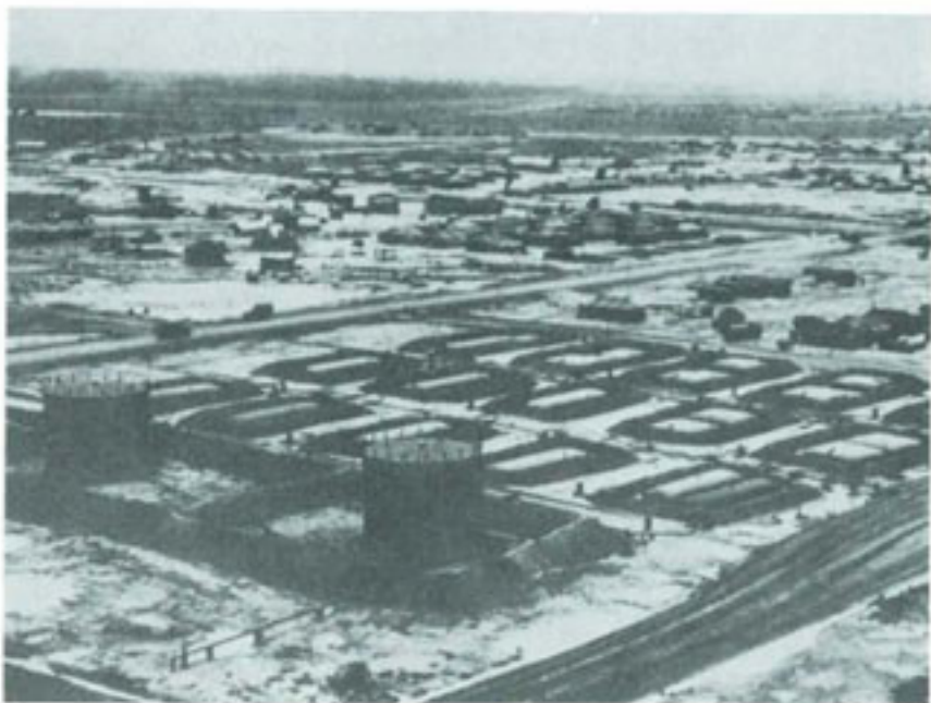
POL STORAGE FARM AT TAY NINH USING BLADDERS FOR STORAGE, ABOVE; LOADING OF CLASS I SUPPLIES FROM DEPOT AT CHOLON, BELOW.
